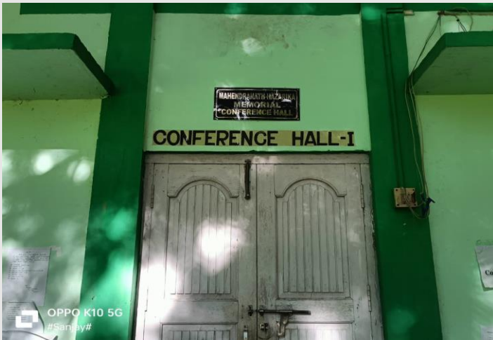
Conference Hall-1 (Mahendranath Hazarika Memorial Conference Hall)
